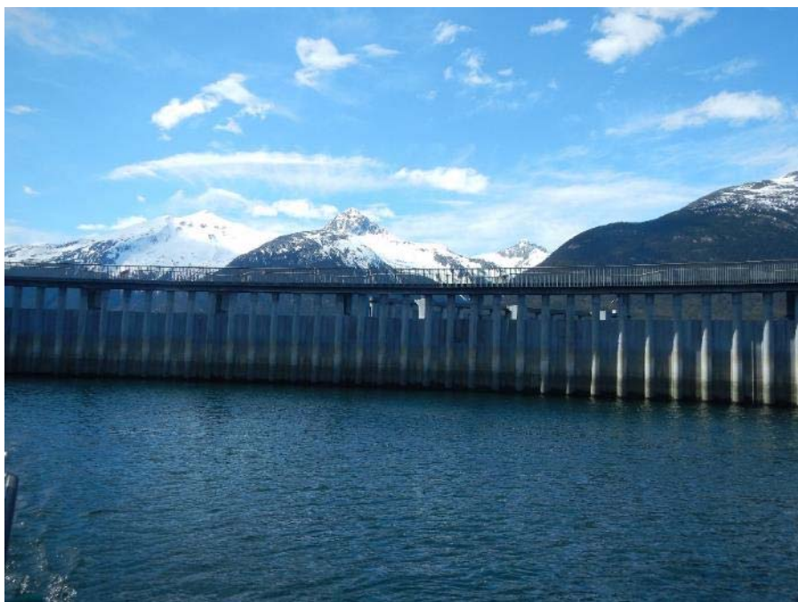
Photo 5: Sheetpile Wall Facing Skagway Small Craft Harbour
