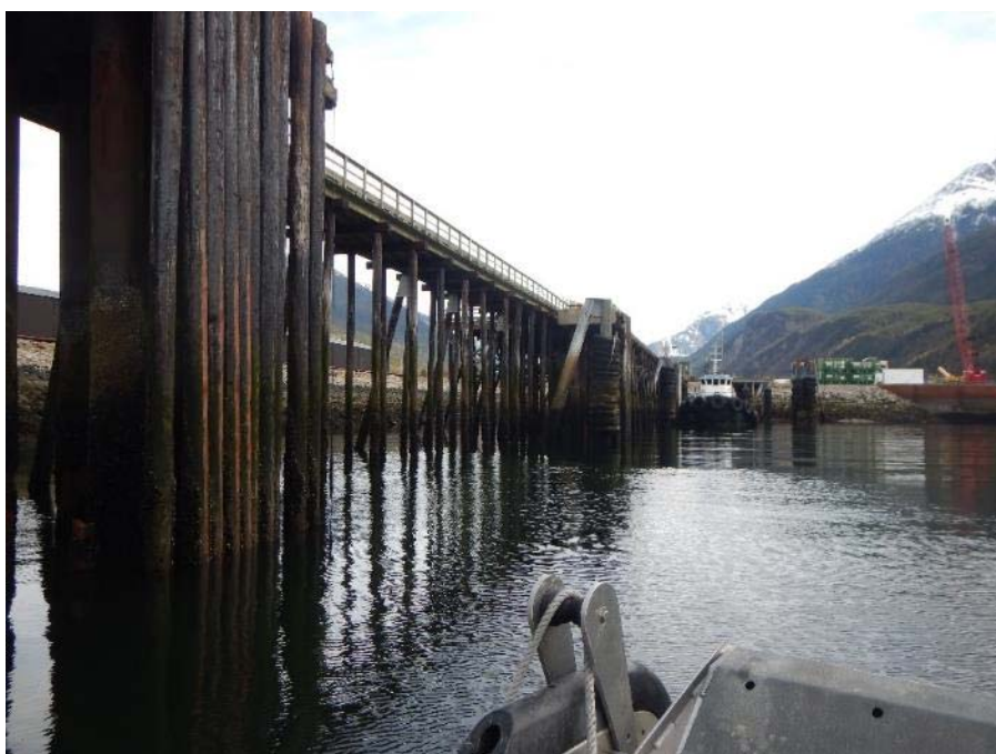
Photo 32: Ore Dock Viewed from SED17-11.
